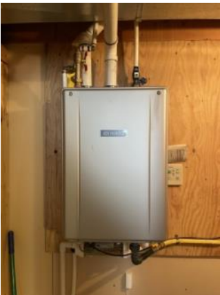
Furnace & hot water on demand unit located in the closet in the basement 3 piece bath. .
