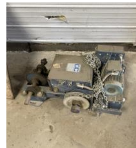
MOTOR LIFT FOR OVERHEAD DOOR (not installed)
