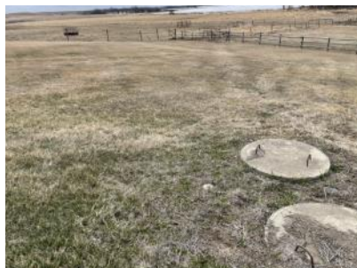
Sewer - tank & field (home)
