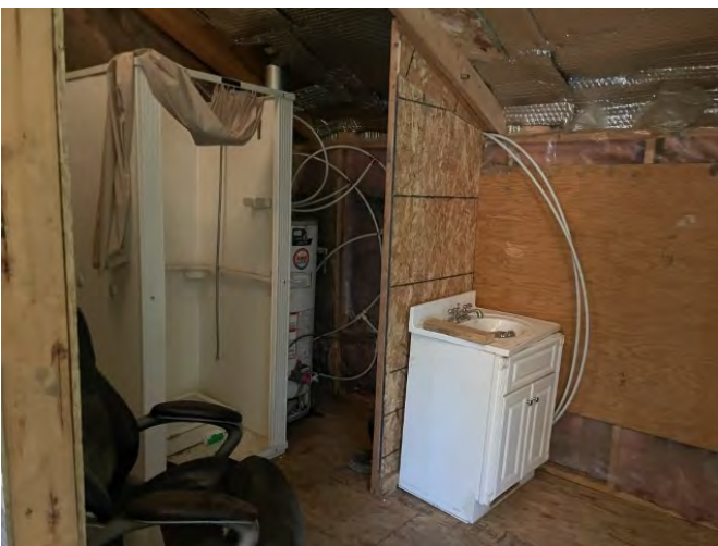
UPSTAIRS - 3 piece bath with water heater that was also used for in-floor heat.
