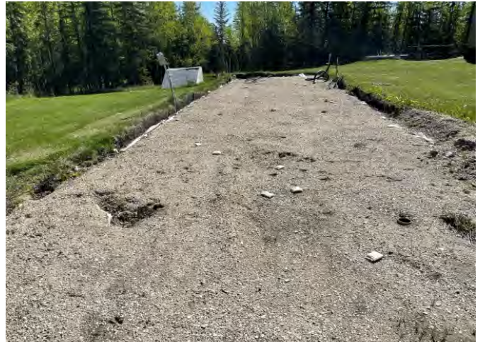
Gravel pad for former mobile home. With sewer, water power and phone line hookups
