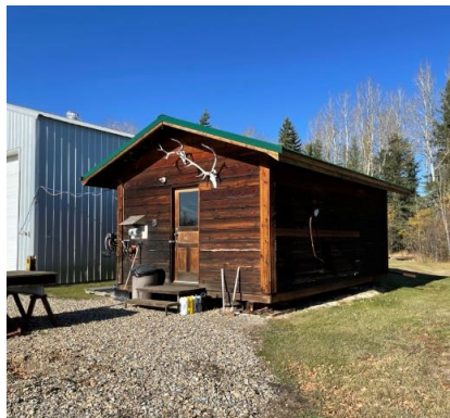
Original 2 room homestead cabin with square timbered construction, metal roof. Power is by extension cord from the shop.
