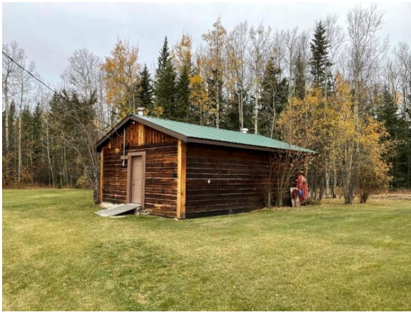
Square timbered construction workshop, power, 220 wiring, OSB flooring, woodstove, metal roof.
