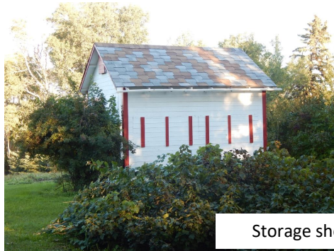
Former garage - used for storage - wood siding, asphalt shingles, power, wood floor. 26'x12'
