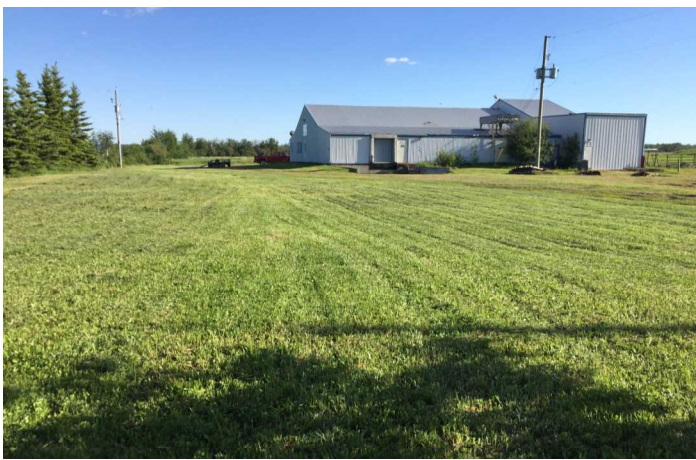
Looking at northwest corner of main building From across the large dugout.
