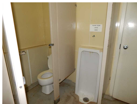
Former mens washroom located in living area
