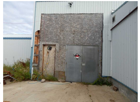
Former overhead door has been closed in.
