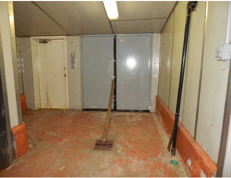
Door to dock
