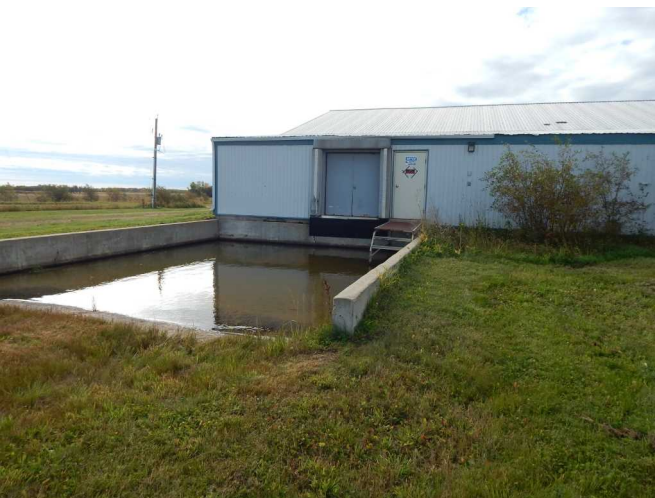
Dock area located on north side of building.
