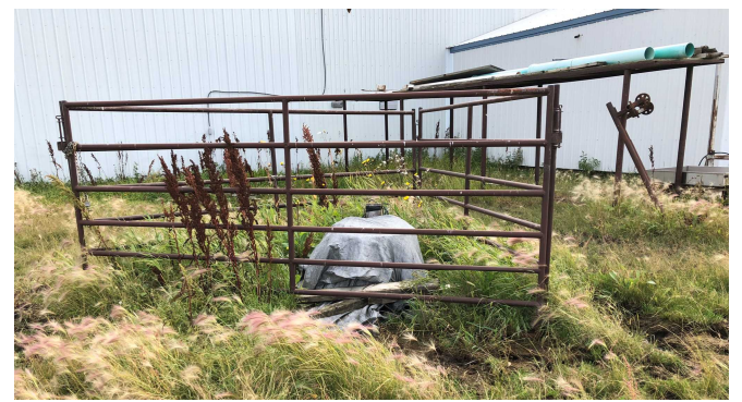
Sewer tanks - sewer discharge is west of building
