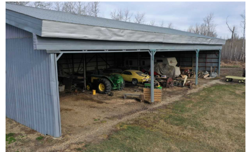
52x80 Solid built pole shed for storage, gravel/dirt floor
