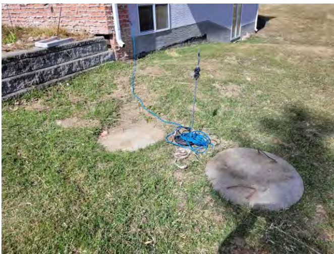
SEPTIC TANKS at corner of home
