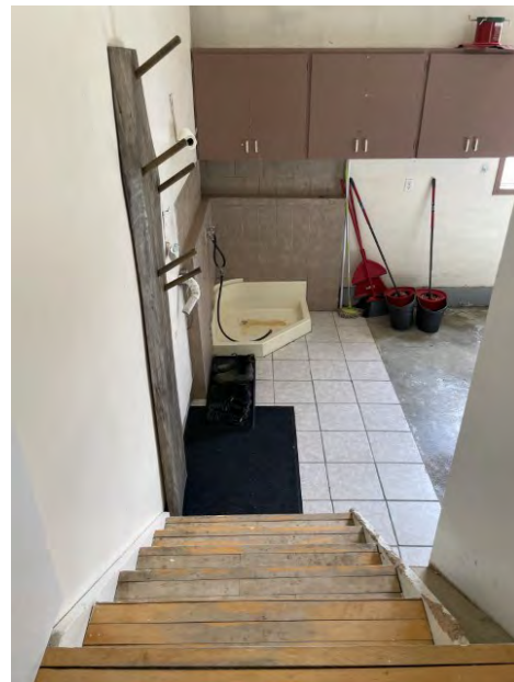
Boot Wash & Stairs down from main floor
